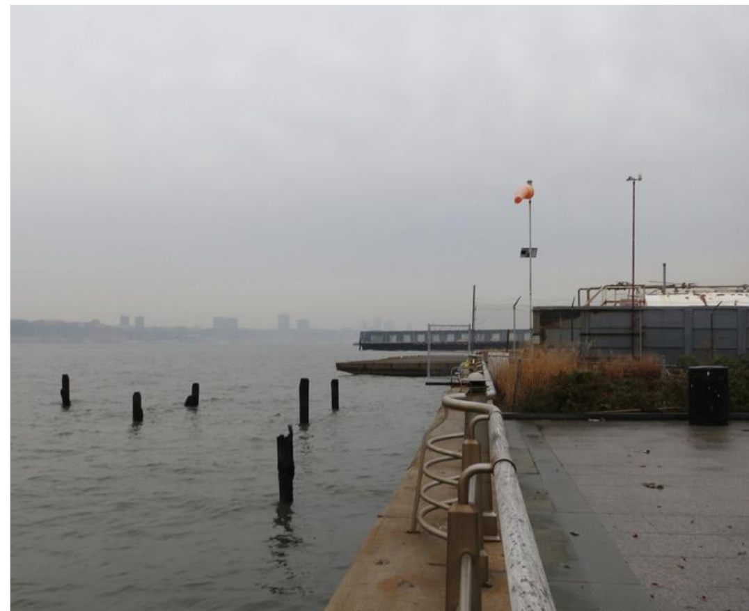
View north of the Hudson River Bulkhead from the foot of West 29 th Street
