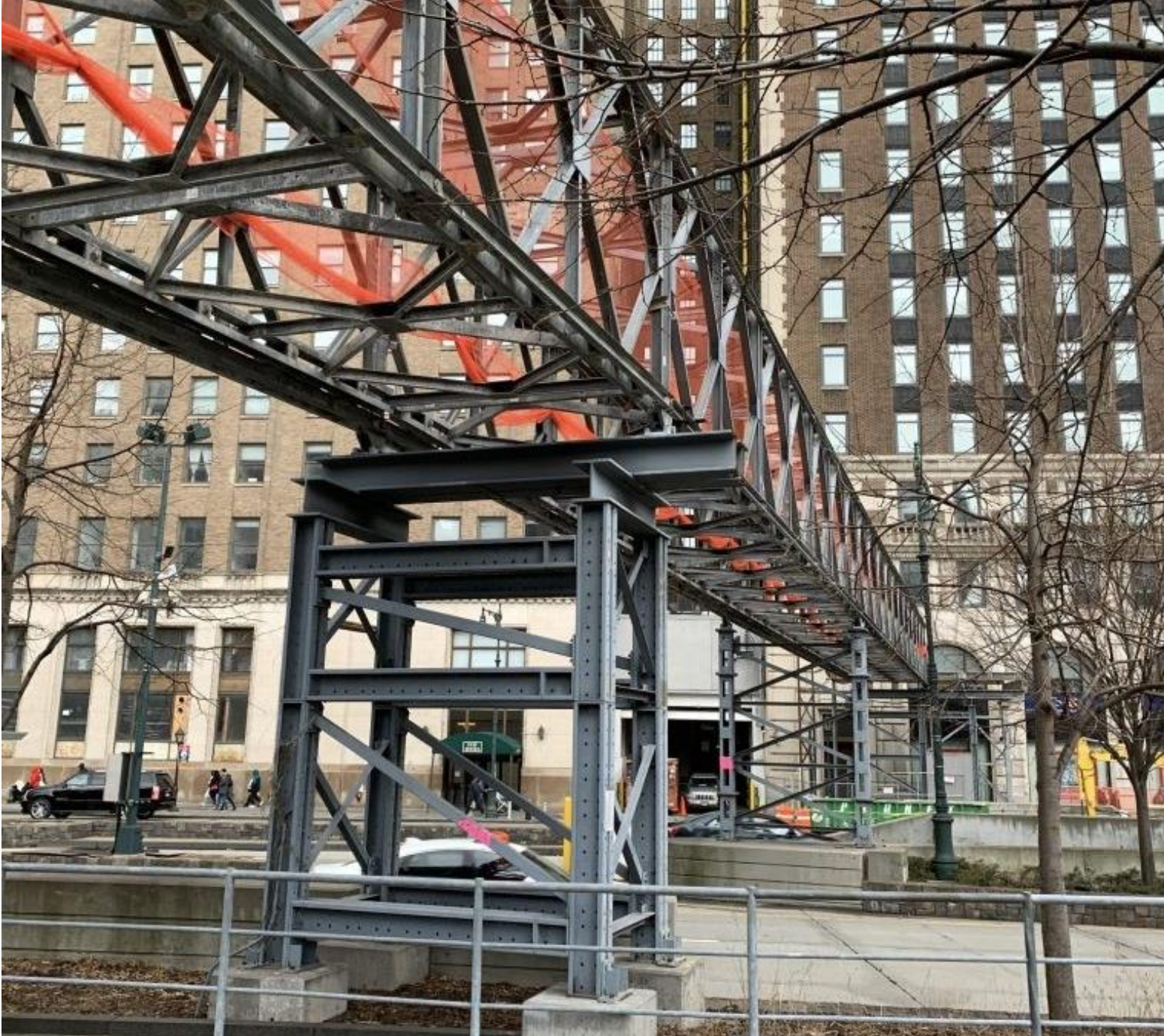
Typical prefabricated utility bridge located across Twelfth Avenue/Route 9A between Carlisle Street and Rector Street
